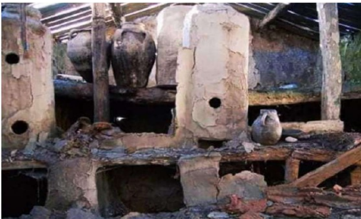
Figure 2: Roofless house (photo by Boualem Rabia)
